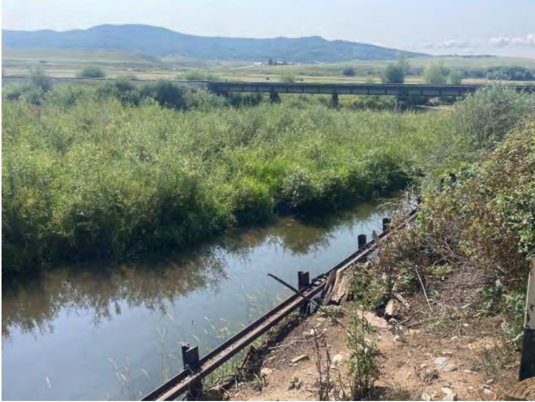
Photo 2: Duquette Ditch return flow (looking downstream)
