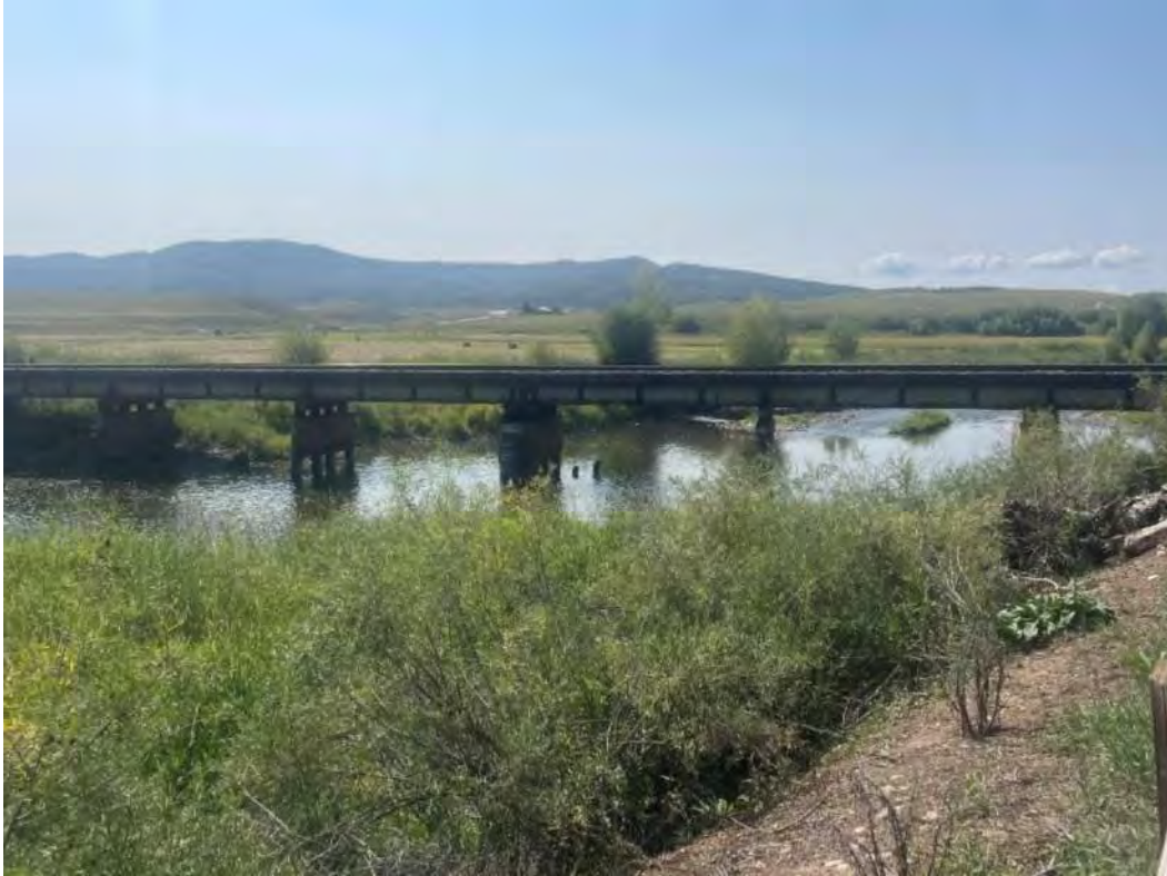
Photo 4: Union Pacific Railroad Bridge (looking downstream)
