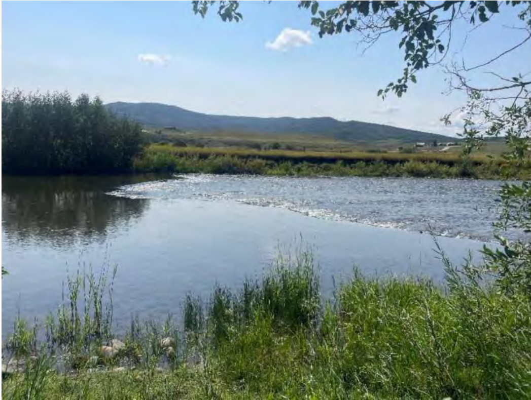
Photo 5: Pushup Riffle for Infiltration Gallery
