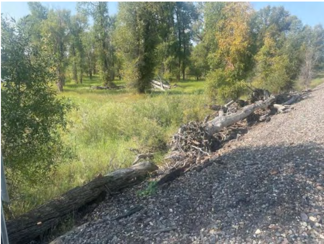
Photo 12: Large wood pulled from railroad bridge abutments
