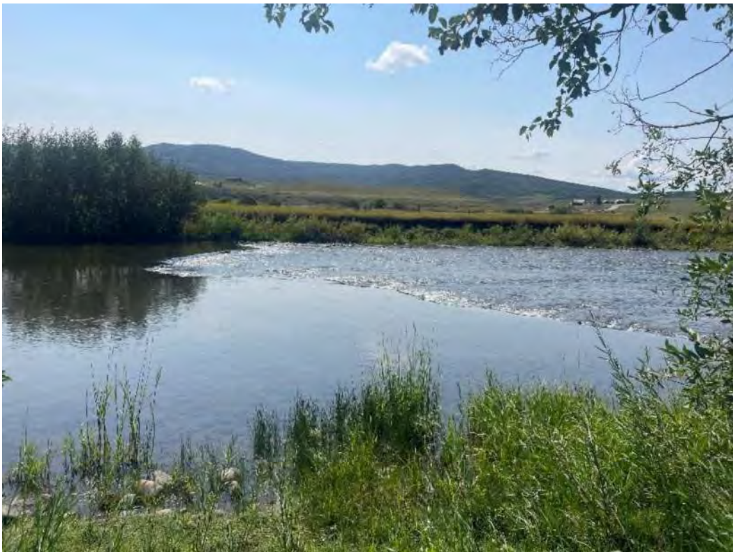
Photo 5: Pushup riffle for infiltration gallery
