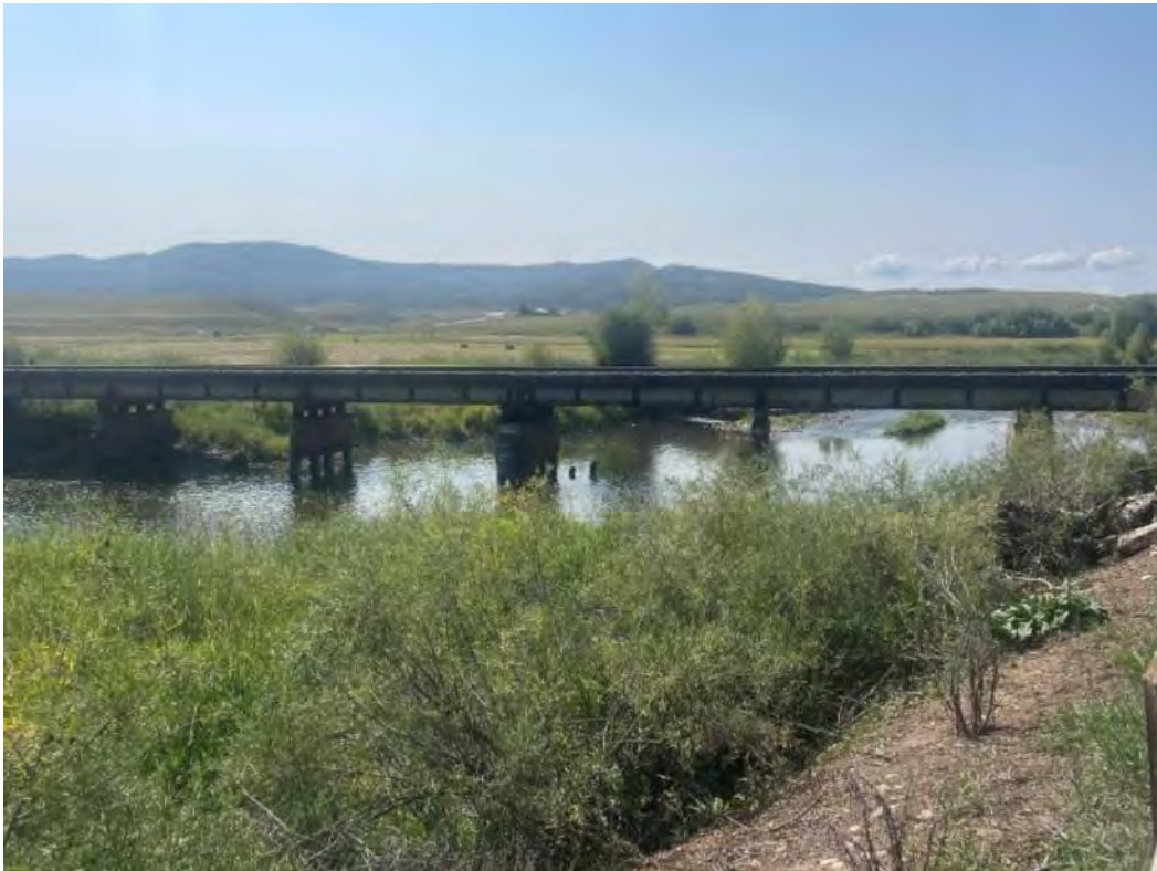
Photo 4: Union Pacific Railroad Bridge (looking downstream)
