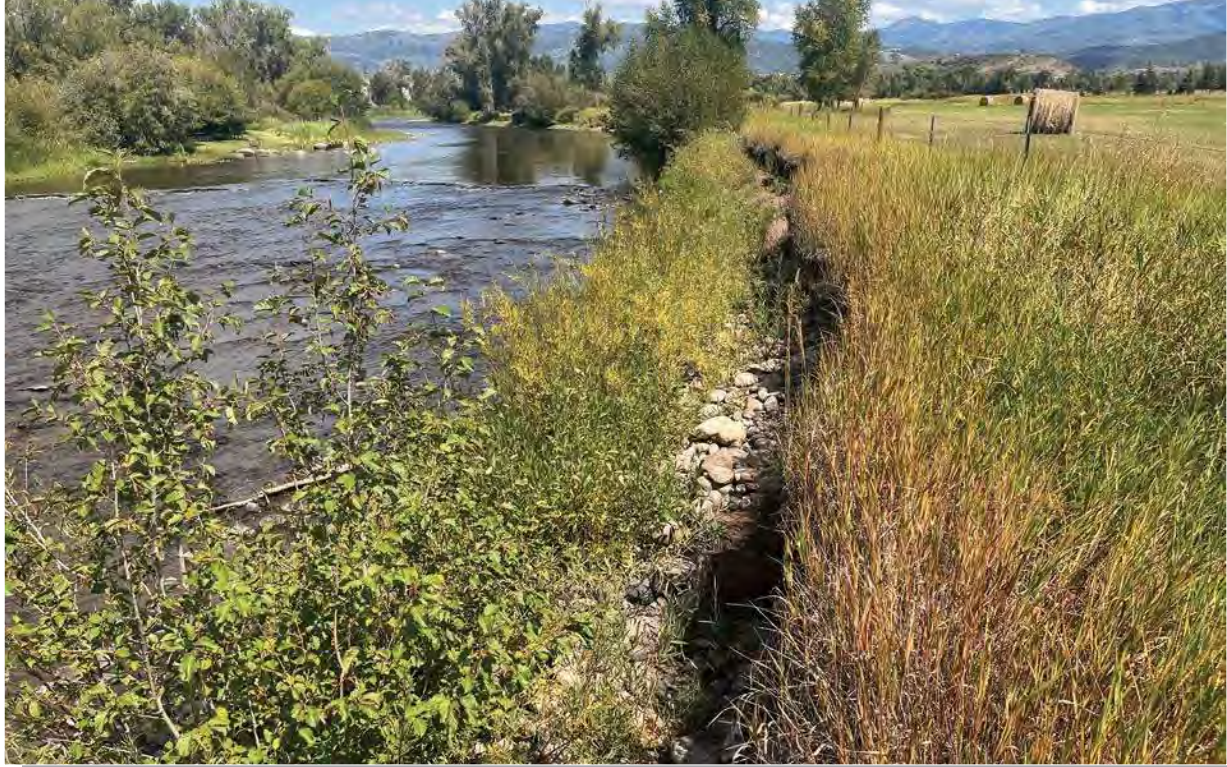
Photo 3 - Prominent erosion and wetland vegetation along the Yampa River. View is to the northeast.
