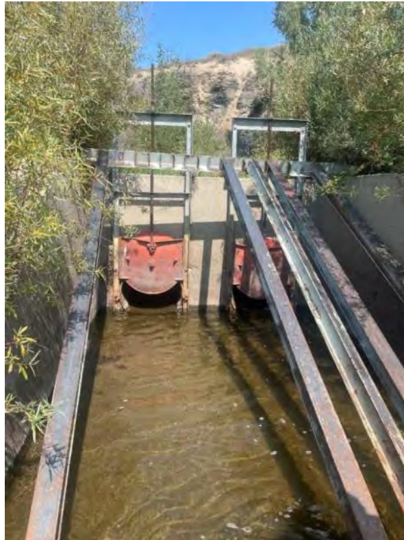
Photo 1: Duquette Ditch headgate
