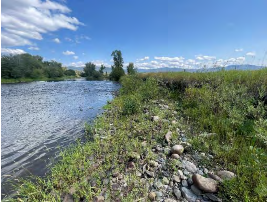
Photo 11: Vegetation establishing at toe of previously failed bank
